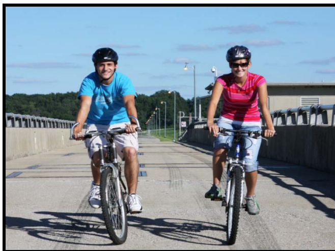
Bicyclists enjoy a scenic view of Carlyle Lake while utilizing the multi-user trail across the Main Dam.
