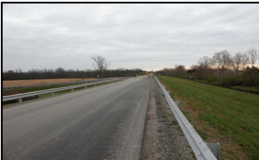
Saddle Dam II road before multi use trail lane was added.
