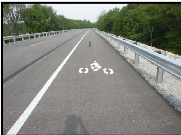
The placement and installation of trail markers along multi-use trail.
